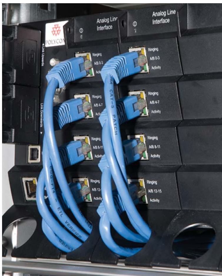
Figure 11 Harnessing cables to the back and out
